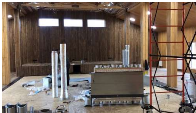
Instalation of air-conditioning and ventilation system in Jagrti building
