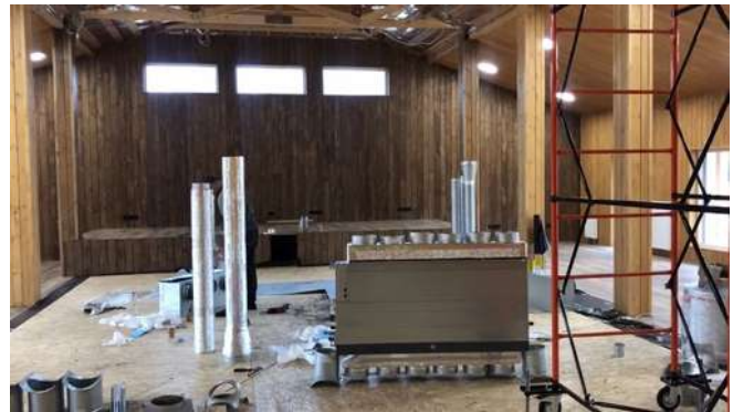
Instalation of air-conditioning and ventilation system in Jagrti building
